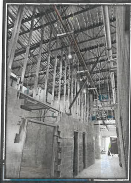
25.08.06 - Area B Metal Framing to Metal Deck
