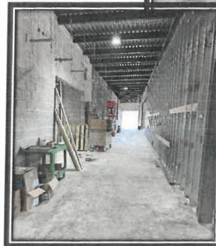
25.08.06 - Corridor Metal Framing Rough-Ins
