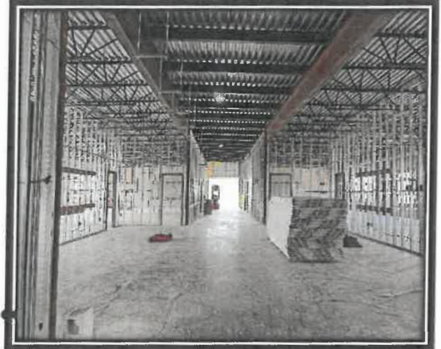
25.08.06 - Area A Metal Framing & Blocking
