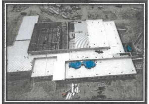
25.06.16 - Areas B/C Structural Steel, Joist & Decking, & Roofing
