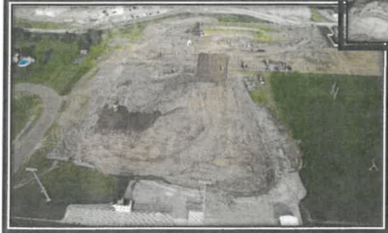
25.06.16 - Strip Topsoil
