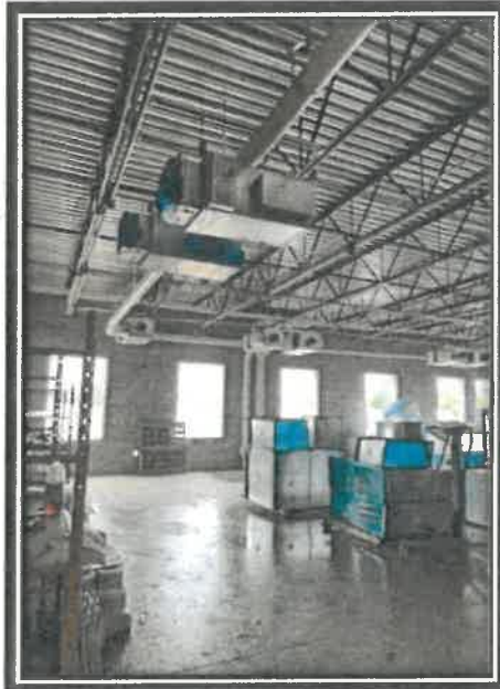
25.06.18 - Area B VAV Installation
