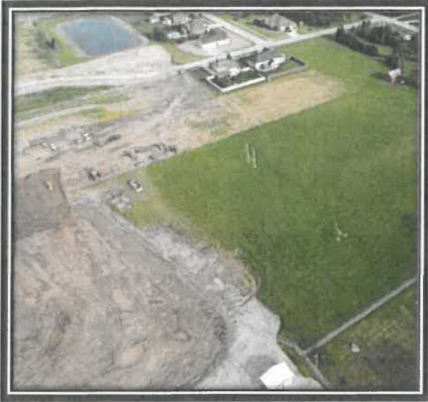
25.06.16 - Strip Topsoil
