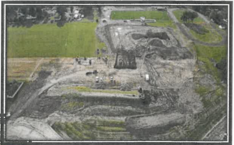
25.06.16 - Strip Topsoil
